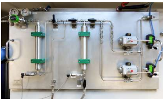
Fig. 3.ac: Bench for testing pressure-regulation piezo valve for ARIANE 6 launcher
